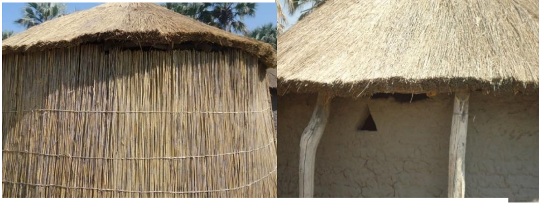
Figure 3: Picture showing eaves in reed and mud hut when used as structural adaptive strategies in mosquito bite prevention by households in the Okavango Delta area (Courtesy: Barbara Ngwenya)
