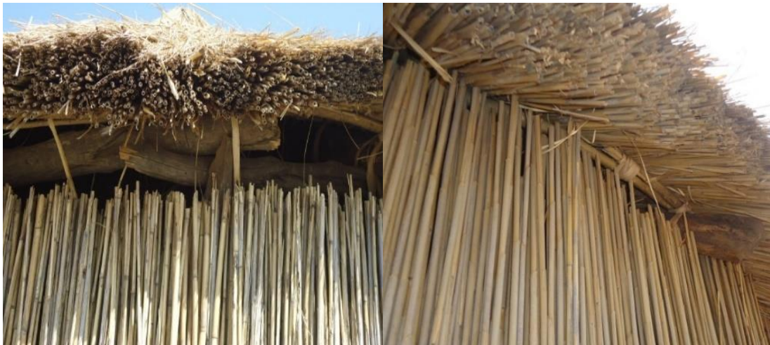
Figure 5: Pictures showing eaves in the reeds when used as in structural adaptive strategy in mosquito bite prevention (Courtesy: Barbara Ngwenya)
